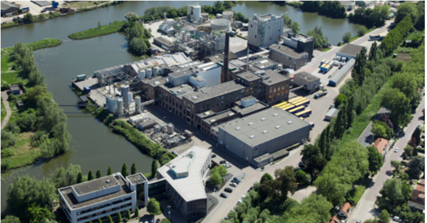
Corbion factory in The Netherlands
